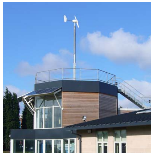
Wind Turbine at Markham Vale Innovation Centre
