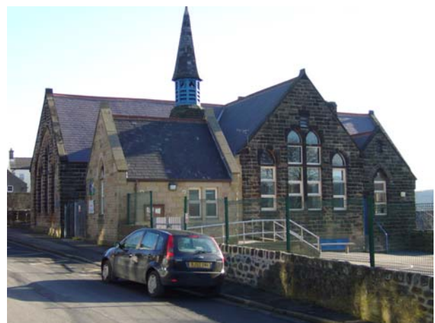
The black fencing at All Saints School, Matlock above is hard to see.
