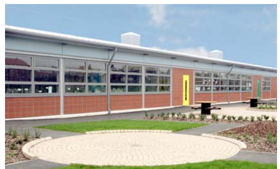
Heanor Mundy Junior School was built on a greenfield site as a replacement for Heanor Junior school.
