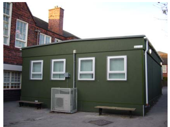
Temporary Classroom at Tibshelf School
