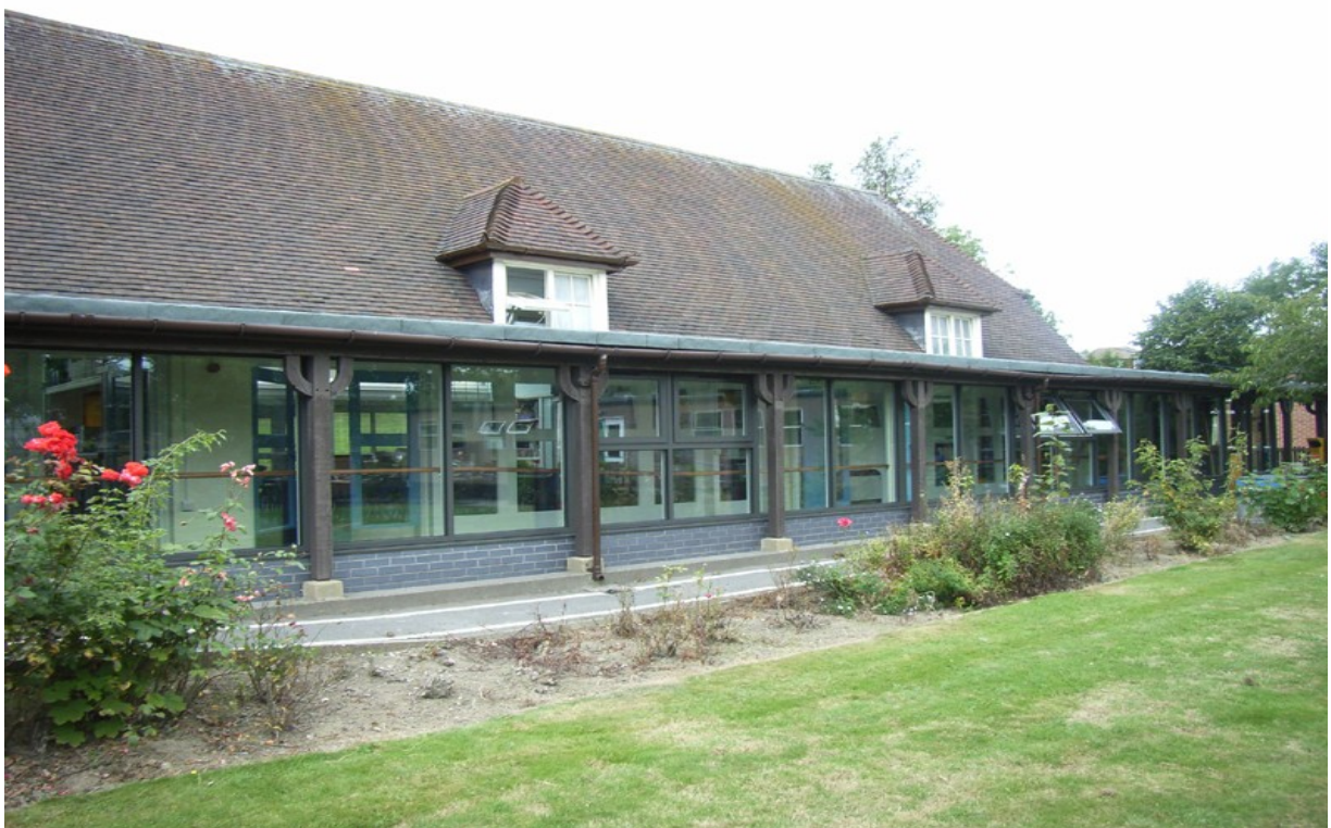
Springfield School, Swadlincote – A typical George Widdows' designed School modernised by enclosing verandas
