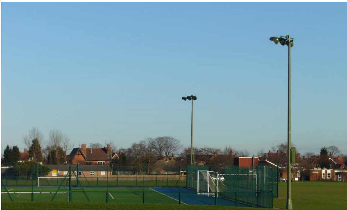
Floodlighting at Willsthorpe School, Long Eaton
