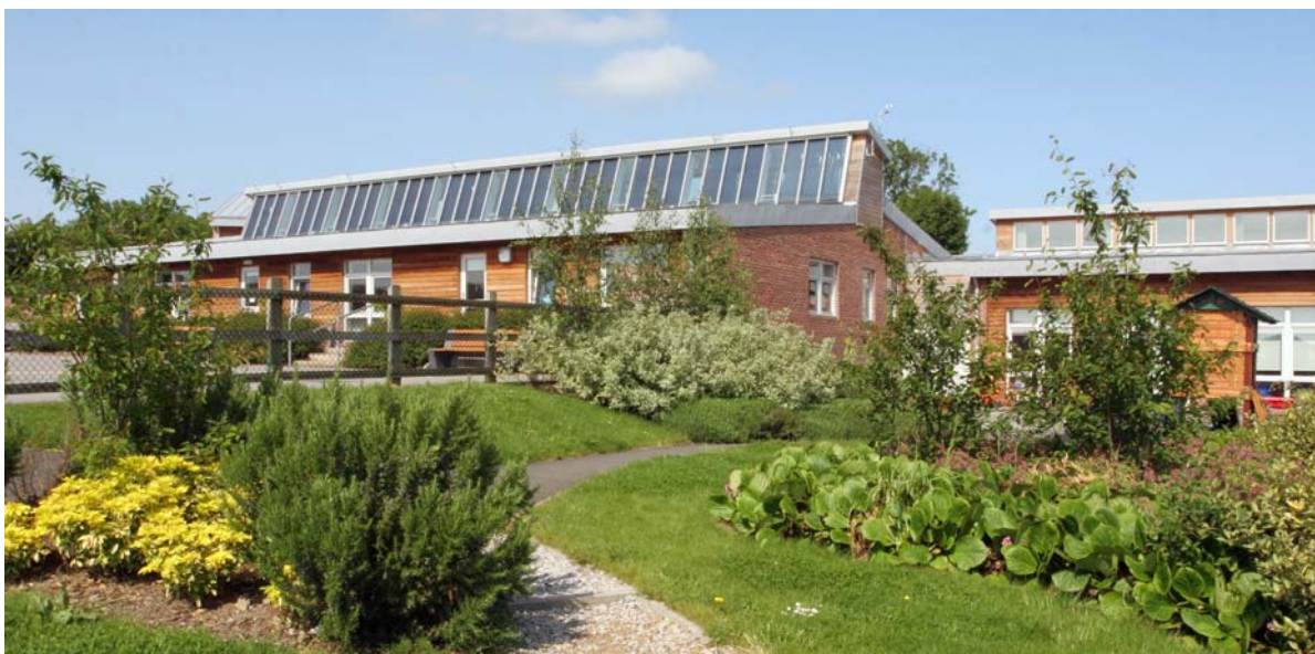
Holymoorside School - windows designed to maximise use of passive solar energy
