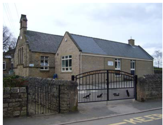
Scarcliffe Infants and Junior School. The relationship of the extension with the existing building is important.
