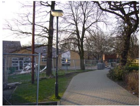
Hasland school. The presence of trees on the site dictated the location of the extension.
